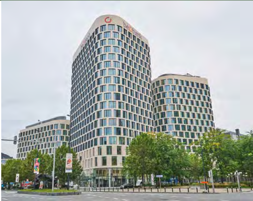
Quatuor Building – SA M. & J.M. Jaspers et J. Eysers & Partners, architectes / architecten.
